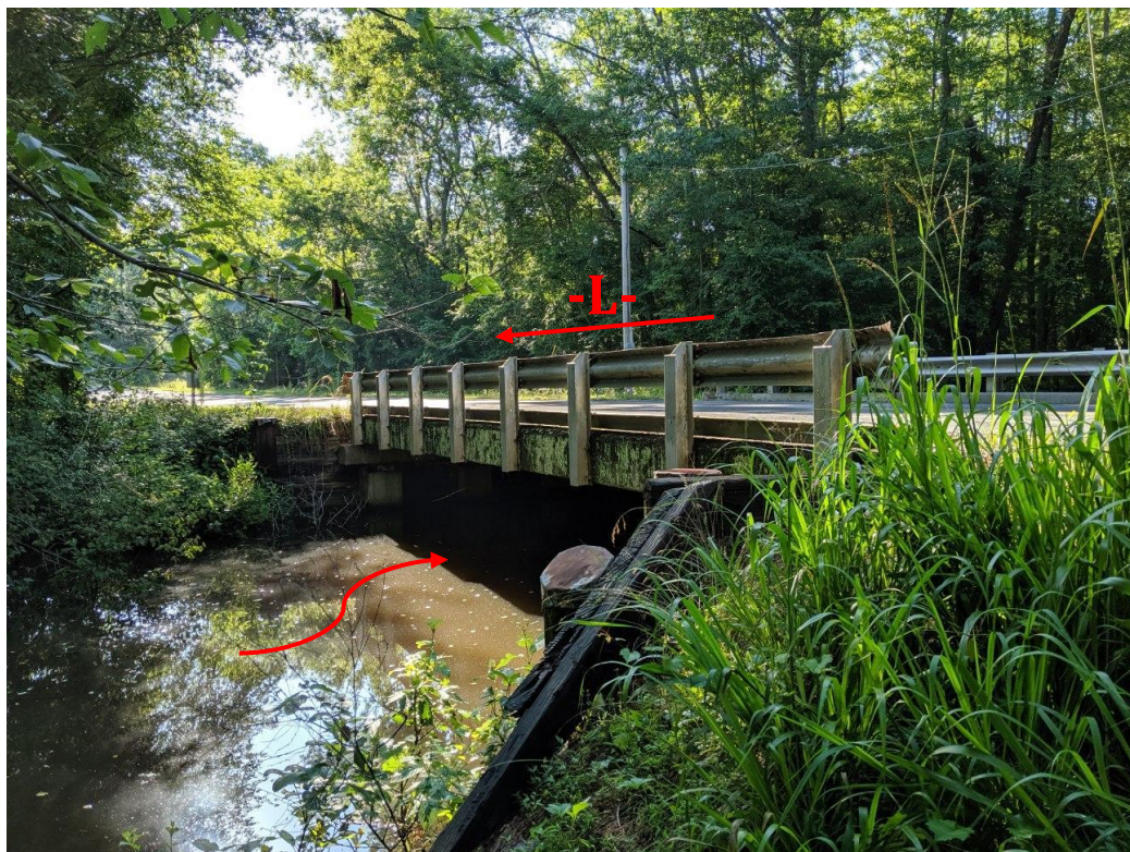
Photograph No. 2: View looking downstream.
